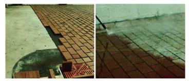
and mortared with a high-bond strength, chemically-resistant polyfurfuryl alcohol-based resin (FURALAC Green Panel Mortar). The room size was approximately 4,500 square feet, with a turnup base being used at room perimeters.
